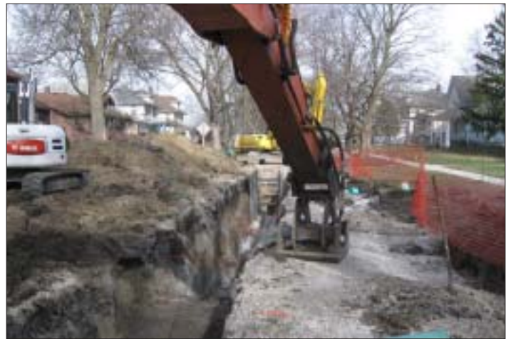
Construction on the Fort Dodge street project.
